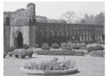
Figure-32: Bara Sona Mosque (Baroduari Mosque) Gaur.
