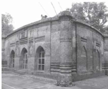
Figure-37: Baba Adamer Mosque, Rampala, Dhaka
