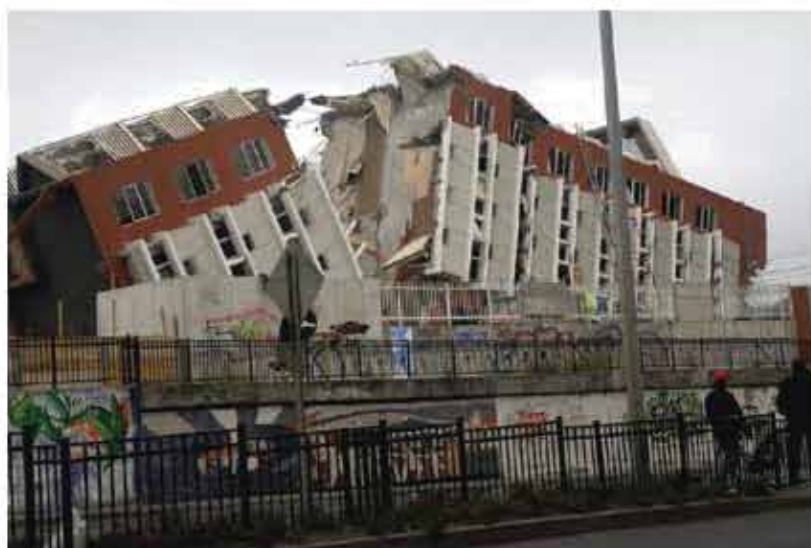
Fig. 9.09 : A damaged building due to earthquake
