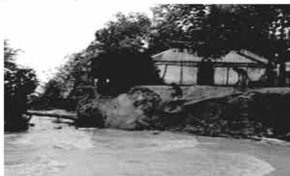
Fig.14.2 : River bank erosion
