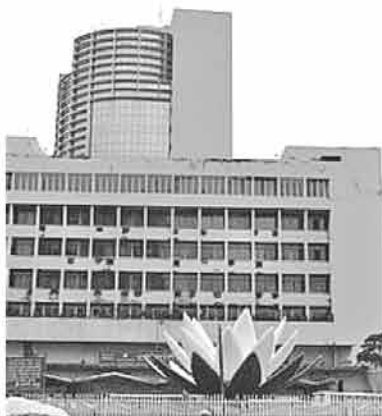
Sonali Bank Building
